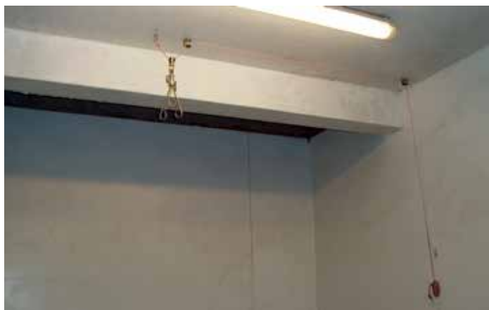
Figure 5. Fluid hangers are hooks attached to the ceiling used for suspending intravenous fluid bags.
