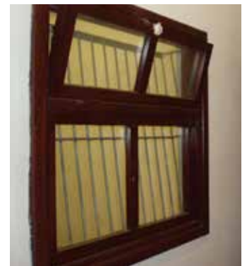
Figure 2. There should be a wire mesh or iron bars covering glass in stables to prevent horses from injuring themselves.
