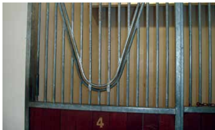
Figure 6. Door grills are used to prevent the horse from being able to get its head over the stable door and damage indwelling intravenous catheters.
